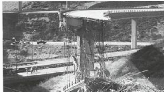
Bridge destroyed by an earthquake.
