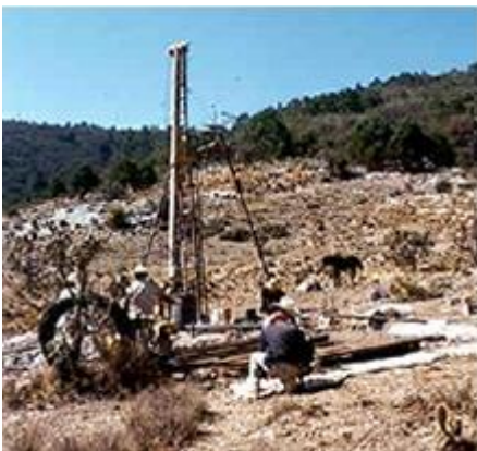
Drilling with diamond bit and recovery of the core
